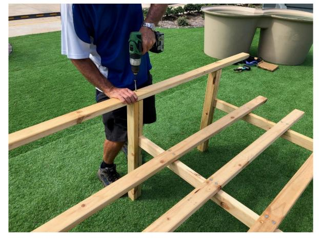
Screw the top frame ends into place as per this image.
