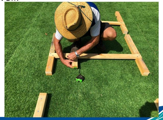
Screw the three support lengths in place as per image (Two screws per joint).
