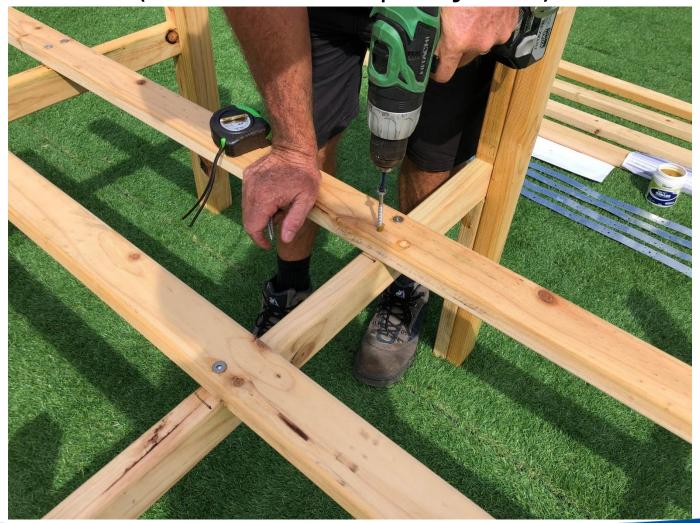
Screw the top/side rails in place using two screws positioned diagonally and into the top of each leg post. The overhang on the ends is 400mm.
