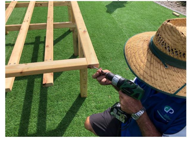
Ensure the legs are upright and the whole frame is square before screwing 1m lengths of bracing into position as per this image.
