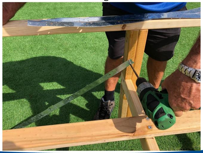
Position the Grow Bed into frame and screw the tub lip to the frame by spacing the small screws provided evenly around the GB800 lip.
